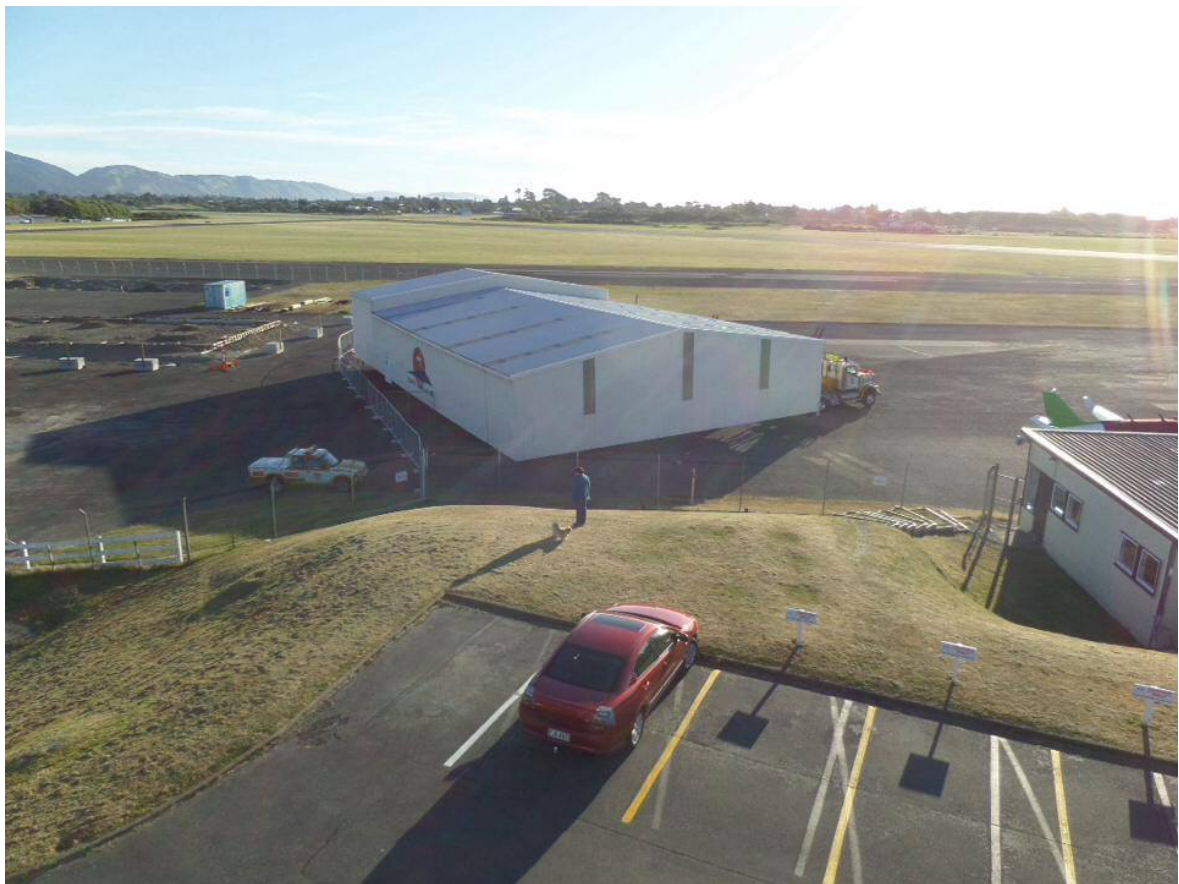
Kapiti Aero Club Hangar being relocated in 2013
