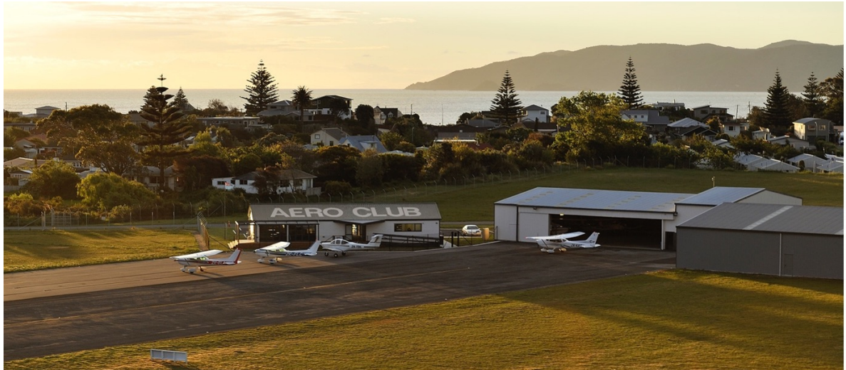
Kapiti Aero Club building and Hangar 2026
